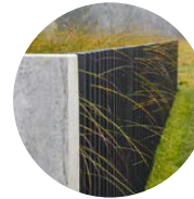
2.1m metal palisade fence
