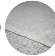
In Situ Concrete
